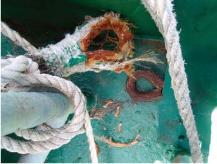
Lifeboat embarkation ladder fixing point condition
