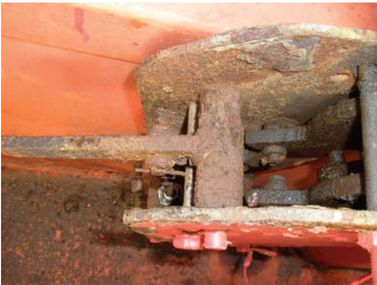
Condition of lifeboat release cables and arrangements
