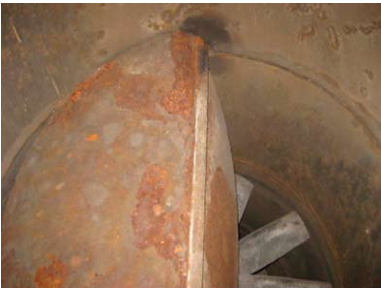
Fire damper condition
