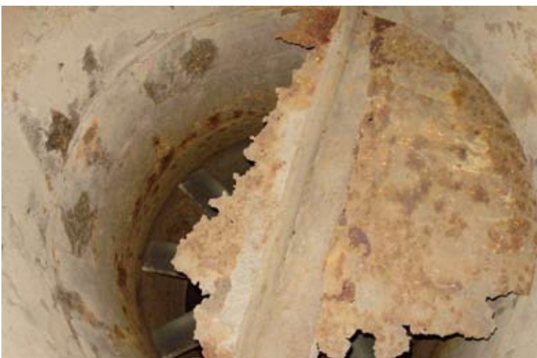
Fire damper condition
