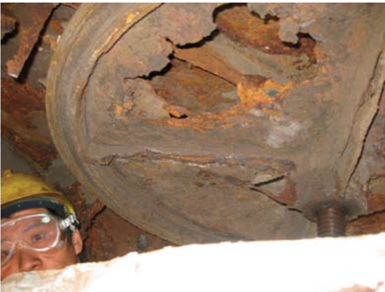
Fire damper condition
