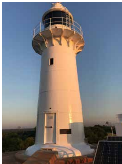
Cape Leveque lighthouse after the 2017–18 paint project
