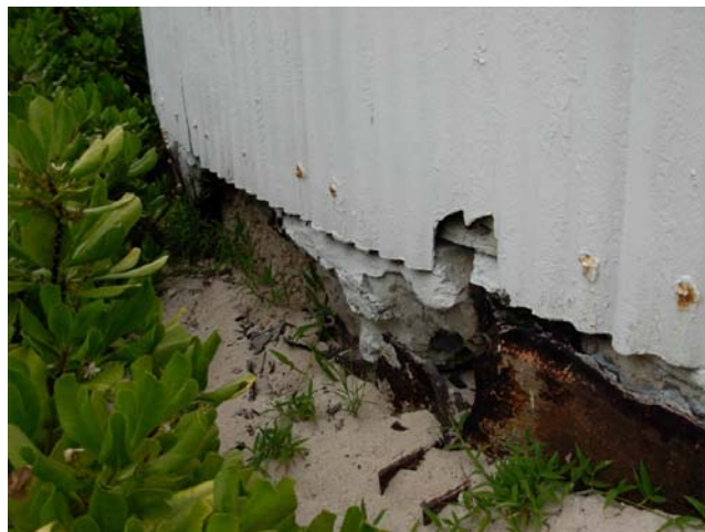
Erosion / corrosion around caisson / foundation
