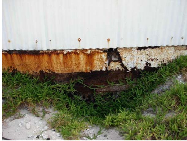
Erosion / corrosion around caisson / foundation
