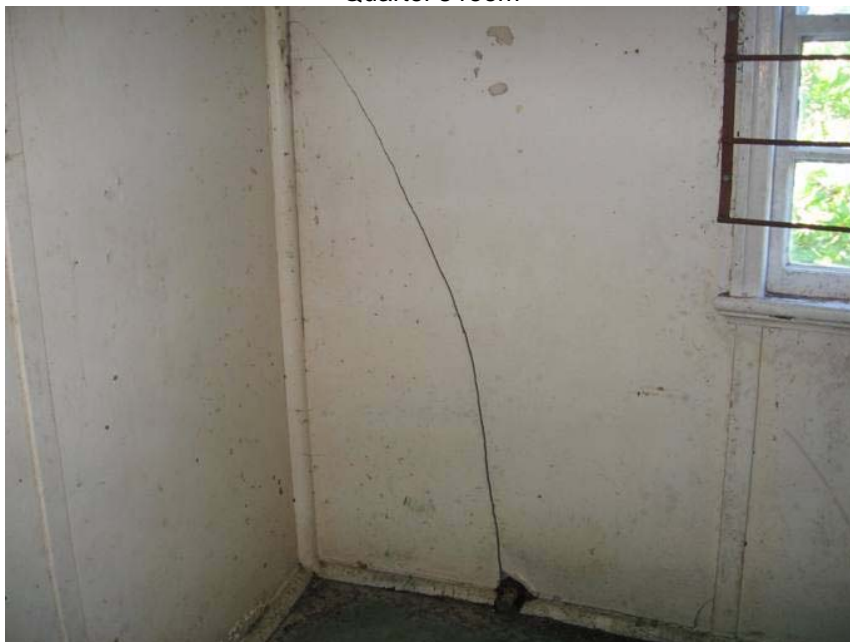
Quarters internal wall sheeting
