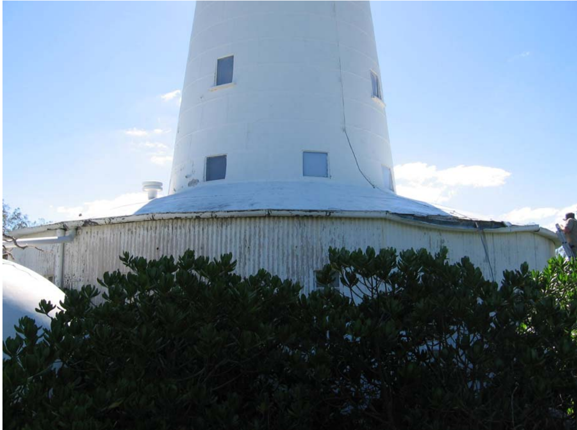
External asbestos corrugated cladding
