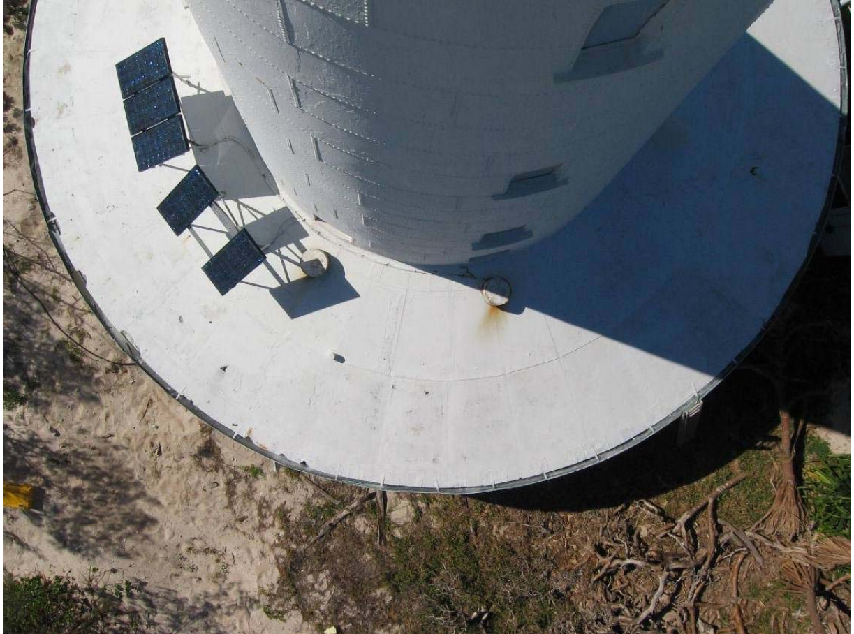
Flat sheet quarters roof
