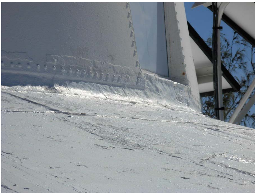
Sealing interface between tower and quarters roof
