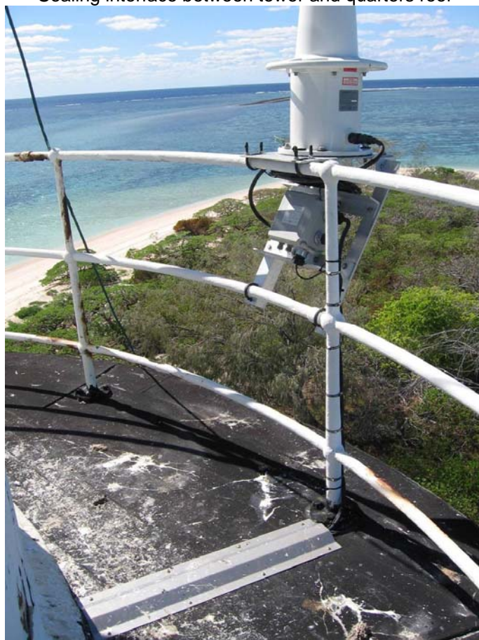
Balcony sealing interface between lantern room and soffit
