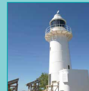
Figure 3. Cape Leveque Lighthouse Photo source: AMMSG 2020
