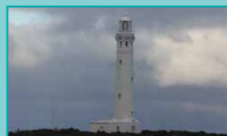
Figure 6. Cape Leveque Lighthouse Photo source: AMMSG 2019
