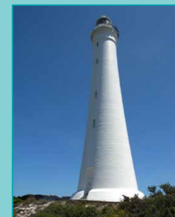
Figure 55. Cape Sorell Lighthouse. Photo source: AMSA, 2012
