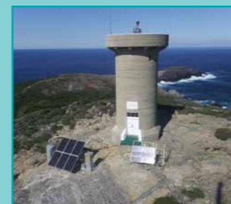
Figure 8. Eclipse Island Lighthouse Photo source: AMSA, 2018
