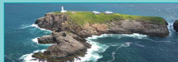
Figure 26. South Solitary Island Lighthouse. Photo source: AMSA, 2010
