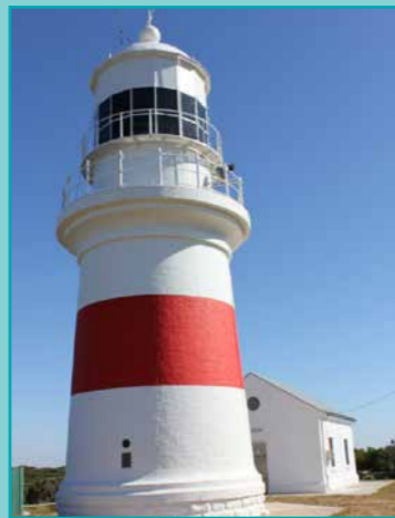
Figure 93. Cape Northumberland Lighthouse. Photo source: AMSA, 2012
