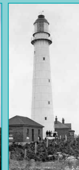
Figure 71. Tasman Island Lighthouse. Photo source: AMSA, 2011
