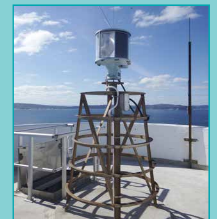
Figure 9. Eclipse Island Lighthouse Photo source: AMSA, 2018
