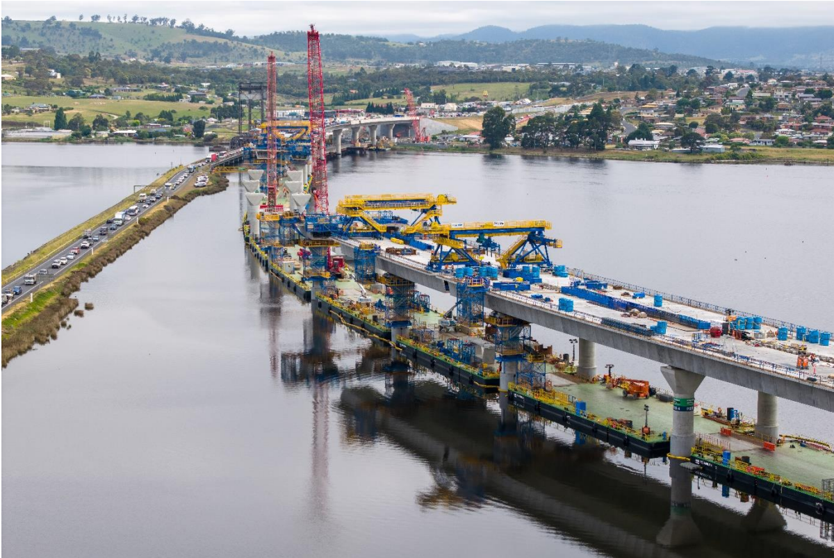
Figure 19 - the 12 NBB barges 12 x 55m spanning the Derwent river
