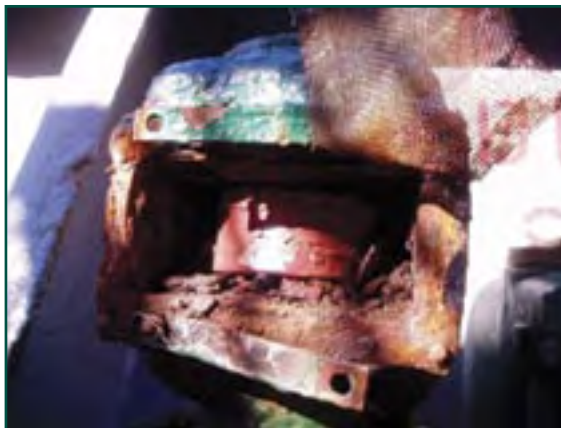
Vent head on deck
