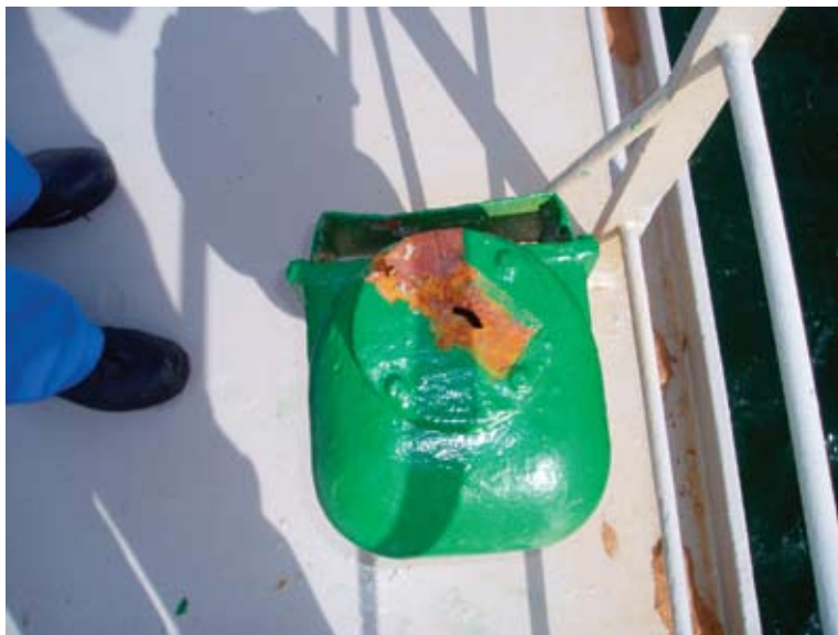
Air pipe taped over and painted
