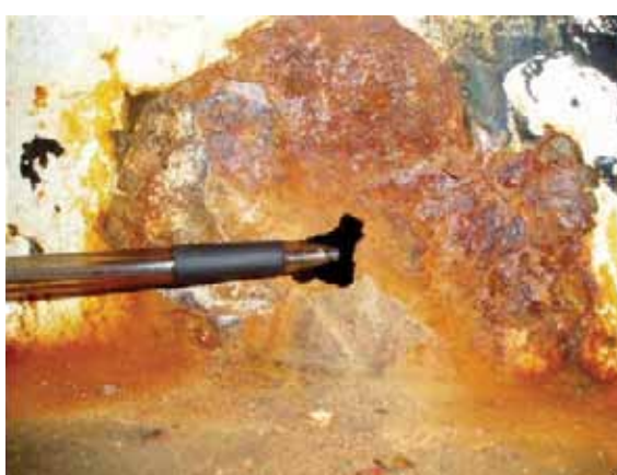
Holed watertight bulkhead
