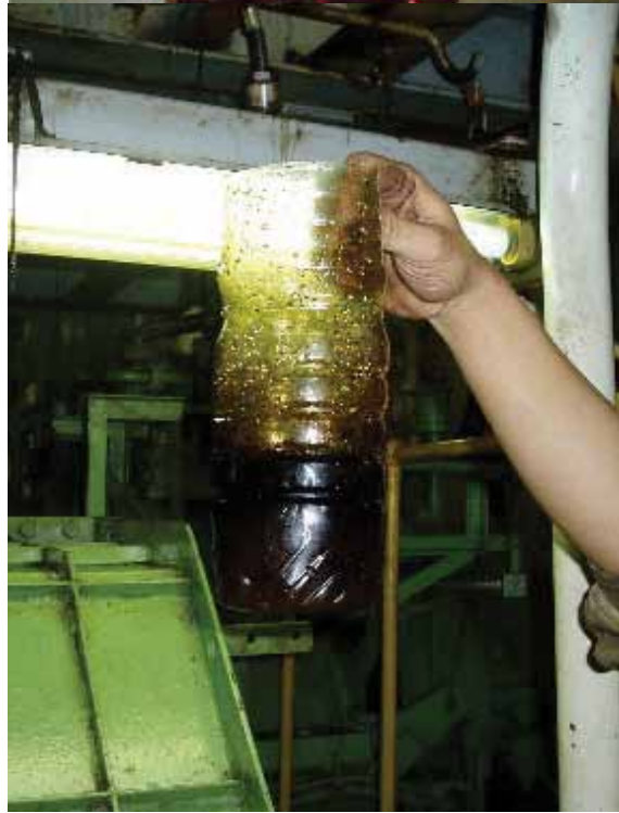
Contaminated water from oily water separator
