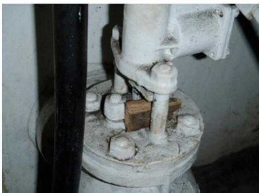
*Service tank valve secured open*
