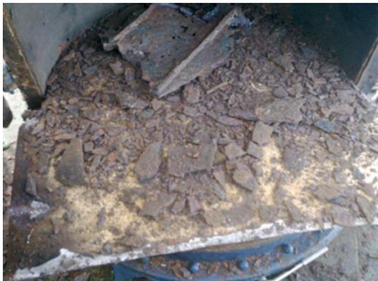
*Collapsed fire damper*
