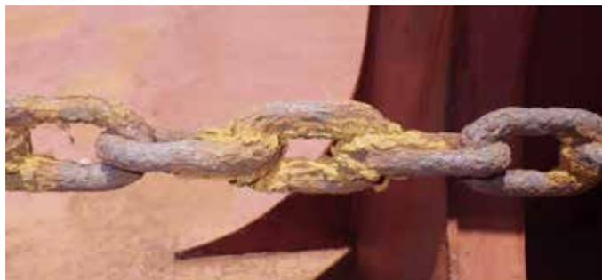
Poor condition of hatch cover chains
