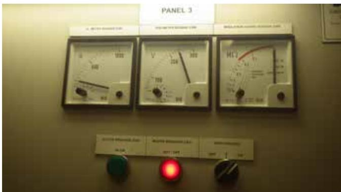
220 Volts Main Switch Board low insulation
