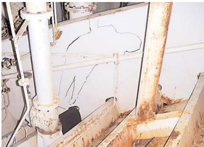
Figure 2: Location of the electrician (source: ATSB)
