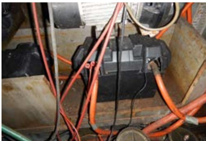
The battery box is not secure and allows possible venting of hydrogen gas to the ignition source on the water pump above.
