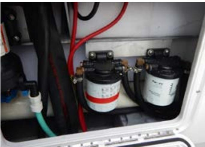
Here, large unsupported wiring is seen running next to fuel filters. Above these filters is a capstan winch, which is a source of ignition and could have ignited the filters and caused an explosion. The filters were subsequently relocated into a compartment that was free of an ignition source.
