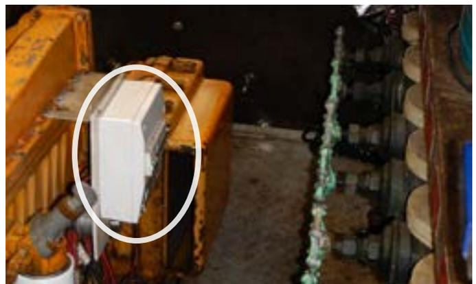
This sub board is unsuitable for its location. There is no cover on the circuit breakers, exposing them to the environment within the engine room, such as people walking past and possible leaks from the manifold directly opposite it.
