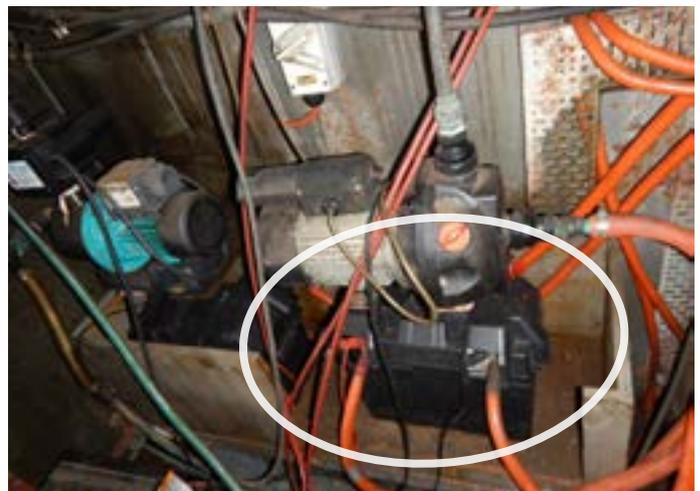
The battery is directly below a source of ignition.
