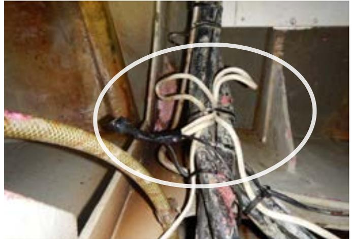
A junction box is required and the wiring needs to be tidied up and secured correctly.
