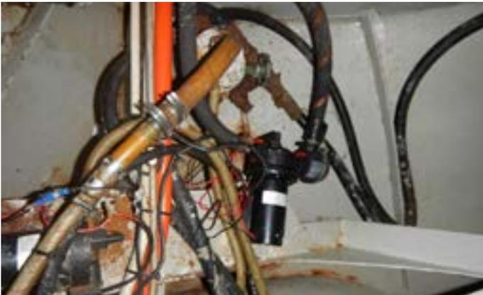
This photo shows untidy, bare conductor terminals. All connections need to be contained within junction boxes.
