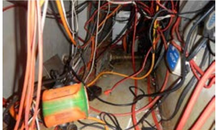
This photo shows unlabelled, unsecured mixed voltage wiring (a mixture of extra low voltage [ELV] and low voltage [LV] wiring) in disarray. In the event of a fault needing investigation, the messy collection of wiring would expose the person carrying out the inspection to the risk of electrocution. Any redundant wiring should be removed to make it easier to find a fault and the remaining wiring needs to be tidied up.
