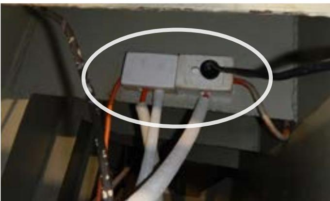
Cable entries need to be completed correctly, and conduits need to be supported to prevent stress on the wiring.
