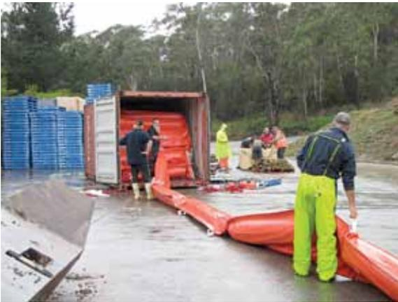
GP Boom from TasPorts, Hobart Tier 1 stockpile being repacked back into container following refloating of the vessel
