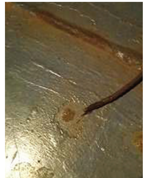
A corroded wire rope on an accommodation ladder, having parted. Source: AMSA Marine notice 13/2014 presentation
