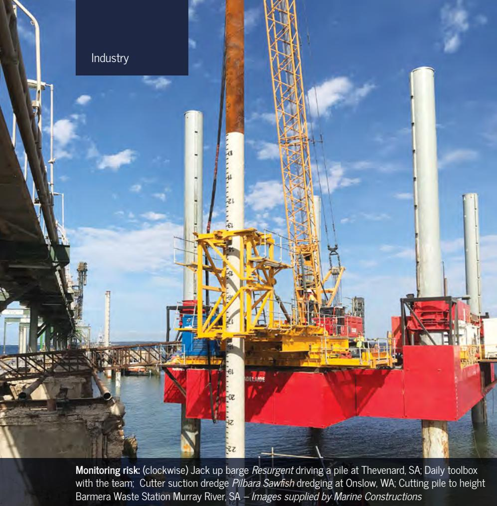
**Monitoring risk:** (clockwise) Jack up barge *Resurgent* driving a pile at Thevenard, SA; Daily toolbox with the team; Cutter suction dredge *Pilbara Sawfish* dredging at Onslow, WA; Cutting pile to height Barmera Waste Station Murray River, SA – Images supplied by Marine Constructions
